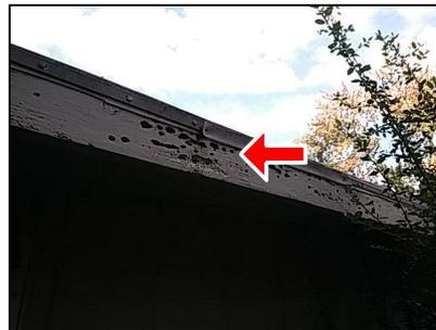
**4.3 Eaves, Soffit, Fascia:** There is a loose area of soffit at the West side of the home that requires additional securing to help prevent pest intrusion.
