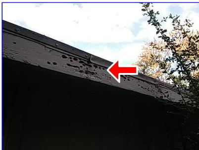
8 **Eaves, Soffit, Fascia:** There is a loose area of soffit at the West side of the home that requires additional securing to help prevent pest intrusion.
