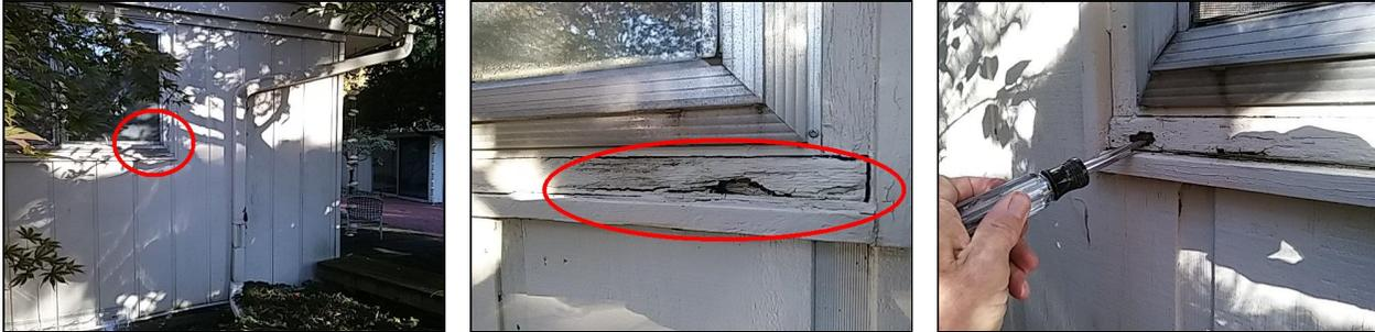
**4.3 Eaves, Soffit, Fascia:** There is some damage to the fascia trim at the South side of the Garage that may be related to past Wood Destroying Organism (WDO) activity. The inspector did not observe any active signs of insects. Repair of the fascia trim will be necessary to prevent damage from moisture intrusion.
