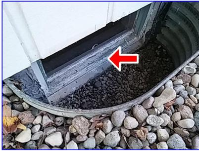
6 **Window Exteriors:** The window sills at the West side of the home are weathered and deteriorated and require repair.
