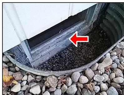
**4.1 Window Exteriors:** The window sills at the West side of the home are weathered and deteriorated and require repair.
