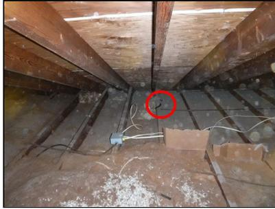
**2.5 Attic Insulation:** The attic floor insulation depth averaged approximately 8 to 10 inches. A more ideal depth for this type of insulation would be about 14-16 inches. As an improvement, you may consider additional insulation in the attic to help with energy conservation, lower humidity levels in the attic, and improved general comfort in the home.
