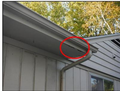
**4.4 Exterior Wall Penetrations:** Exterior wall penetration had gaps that should be sealed to prevent moisture and pest intrusion.
